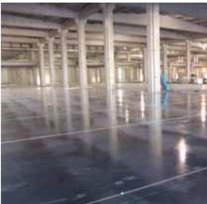
The floor of the distribution centre, belonging to a well known supermarket chain Masoutis S.A. in Greece, was built by Eurolit using Laser Screed construction to meet at least with Line 4 of the DIN 18202 – the strictest DIN free movement specification. CG's involvement in the project was to use their patented Laser Grinder® technology to grind the narrow aisles to a tolerance suitable for the VNA
