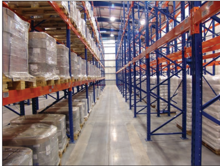
Just after the completion of the racking installation.
